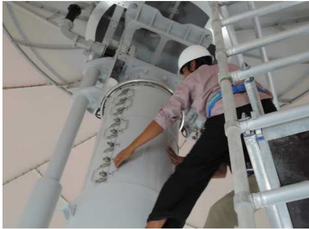
Open the Cover of the Slip ring & Brush (Front Side)
